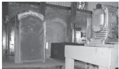
Fig. 3b : Cake charging at Pilot Coke Oven
